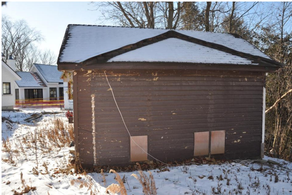
4.4.4.B – Existing Accessory Building B – North Elevation
