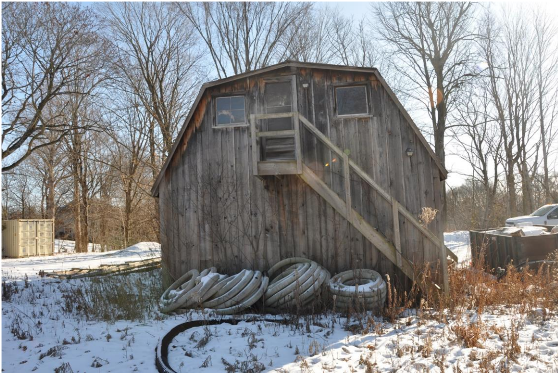
4.4.3.C - Existing Accessory Building A – North Elevation
