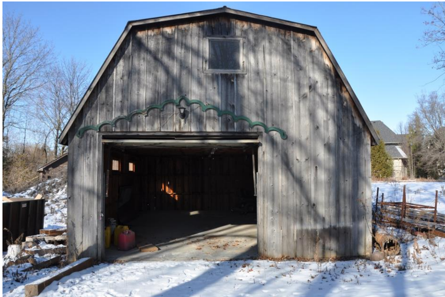
4.4.3.A – Existing Accessory Building A – South Elevation
