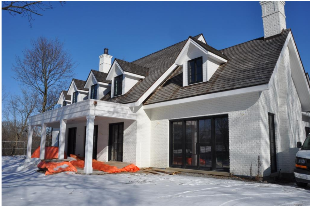
4.4.1.B – Existing Home – Front Elevation view from southwest
