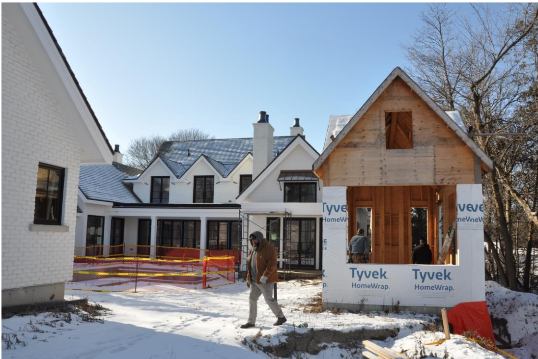
4.4.1.D - Existing Home – Rear (East) Elevation
