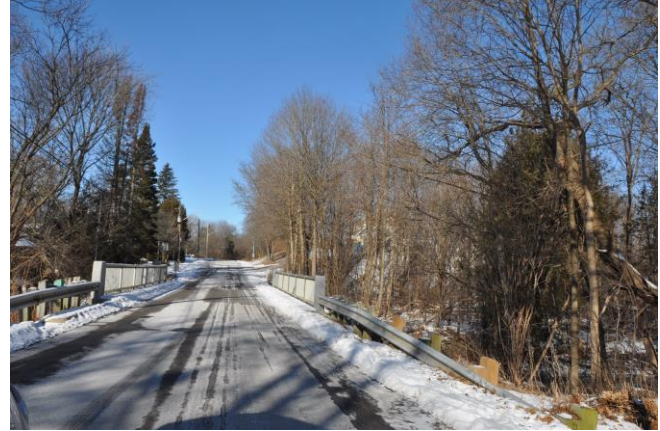
4.4.B - Approach from south
