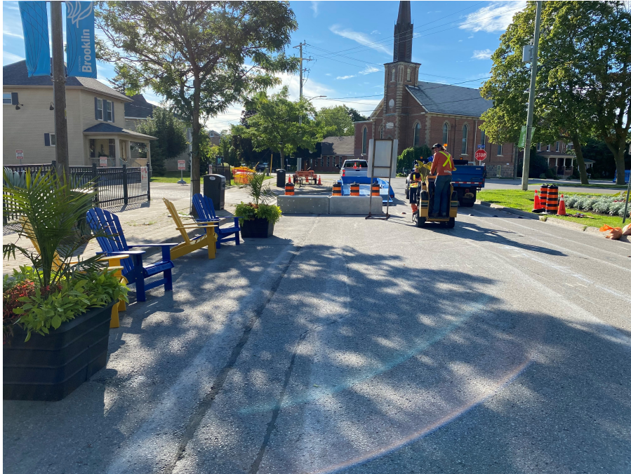
Figure 1 – Installation of Planters and Muskoka Chairs
