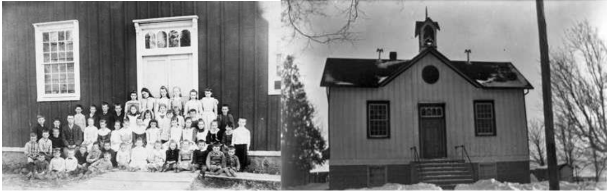
(Left) Class photo c. 1890 at Myrtle School. (Right) View of the school in 1940 after a basement and front stairs were added. The school had a board and batten finish and twelve-over-twelve sash.
