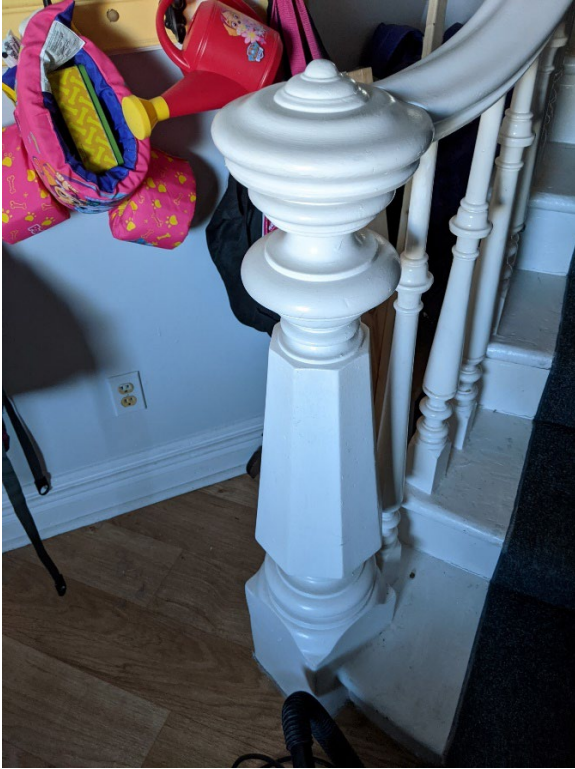
Figure 21: Detailed view of newel post and newel cap (CY 2020).
