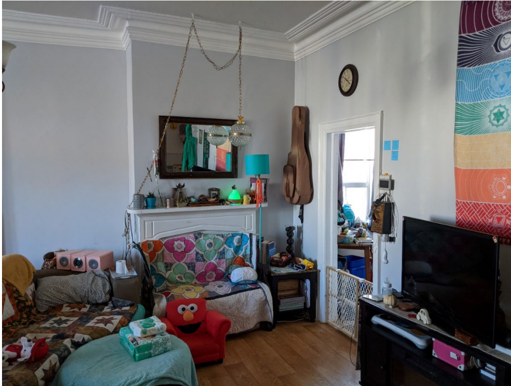
Figure 17: View of first floor room showing interior door casing, crown moulding and fireplace mantel (CY 2020).
