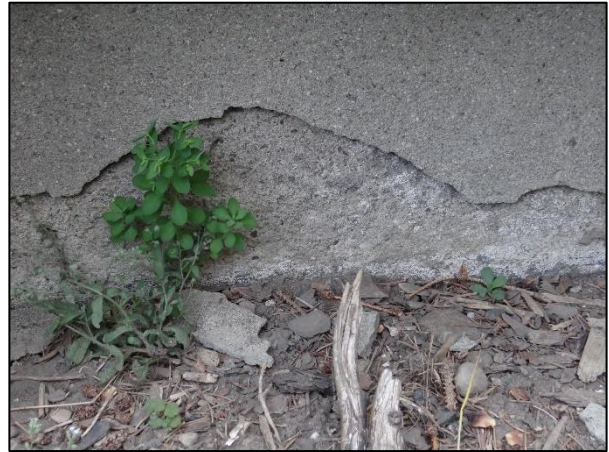
Figure 17: Spalled concrete foundation
