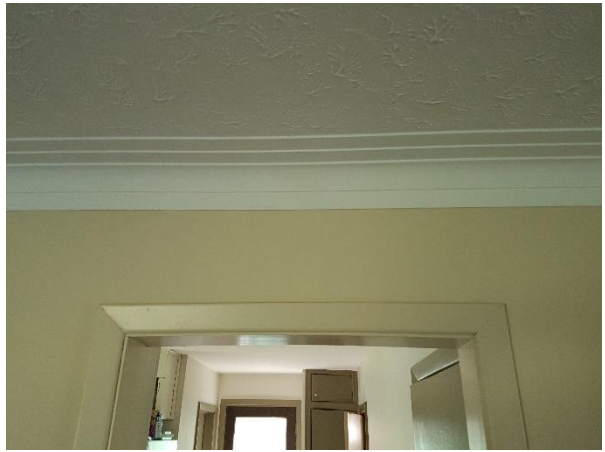
Figure 25: Mouldings and stucco ceiling detail
