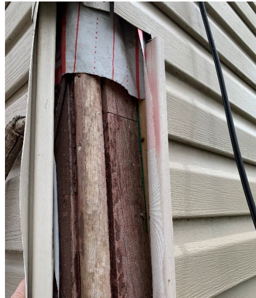
Fig.12: The original wood cladding (MHBC, 2022)
