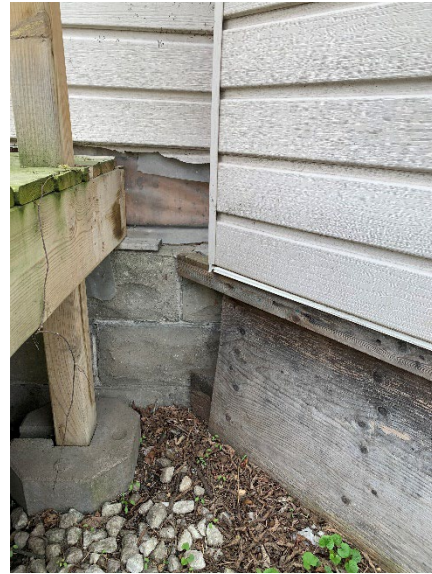
Fig.14: Bay window without foundation (MHBC, 2022)
