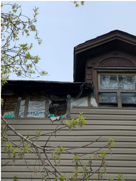
Fig.11: Dormer on side elevation with original bubble glass and wood detailing and shingles (MHBC, 2022)
