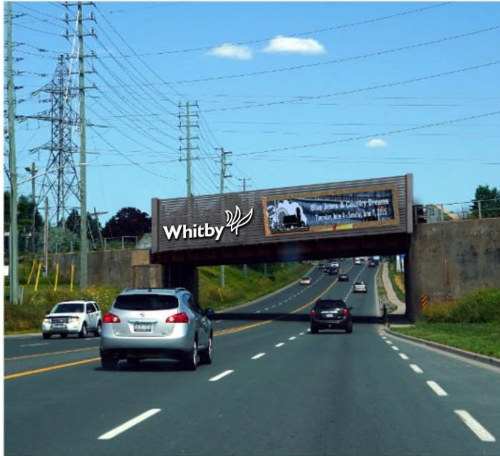
Thickson Road South north of Highway 401 – facing north
