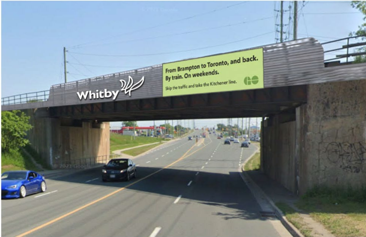
Thickson Road South north of Highway 401 – facing south
