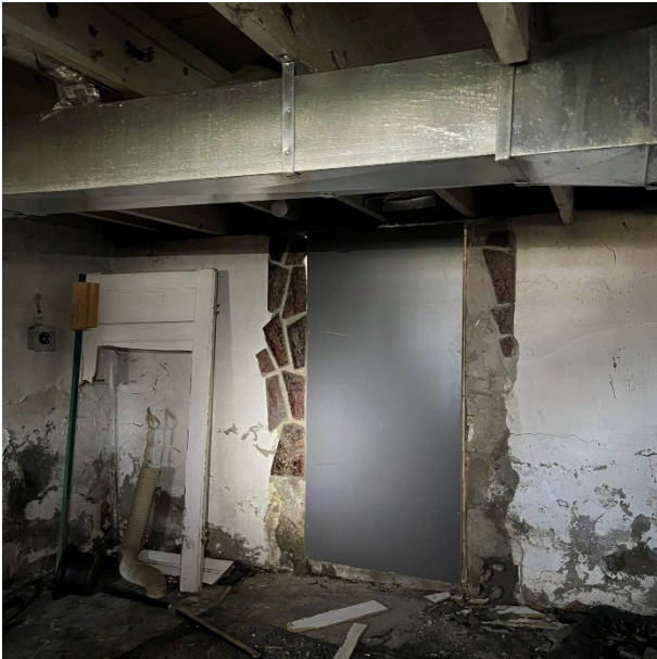
Closed Basement Entrance to Yard
