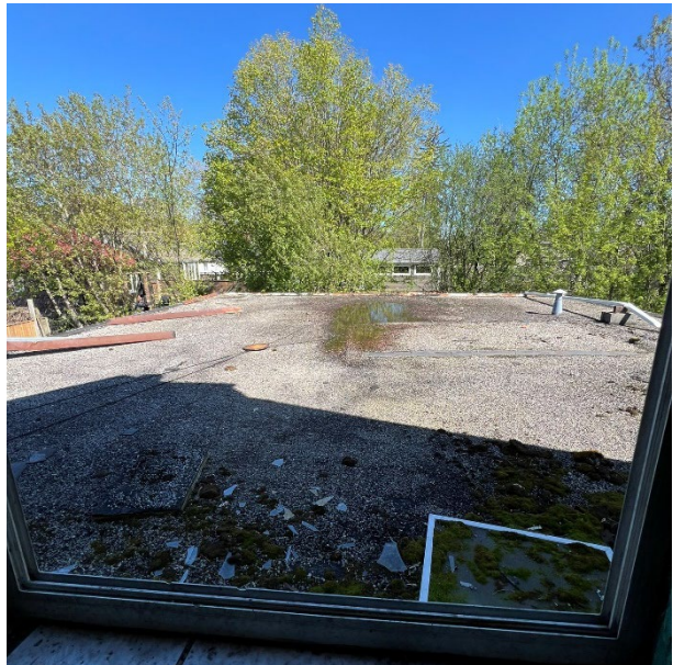
Upper-Level View of Addition
