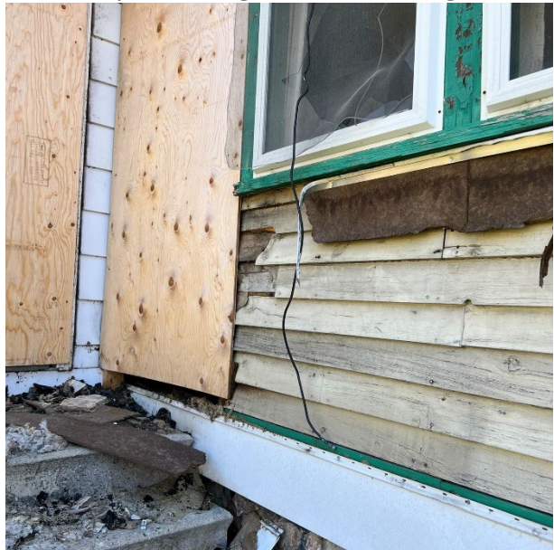
Exposed Original Wood Siding
