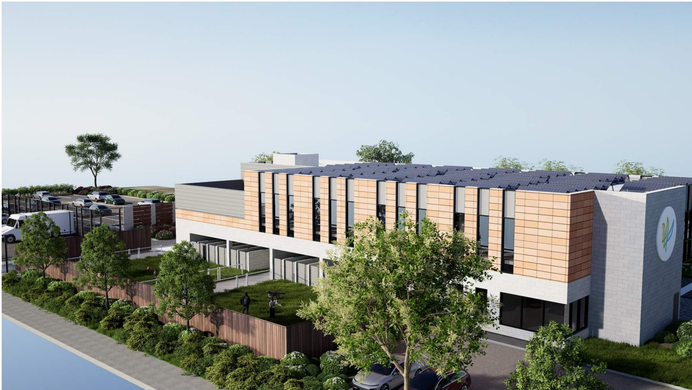
VIEW FROM ABOVE LOOKING NORTHWEST TOWARD THE BUILDING
